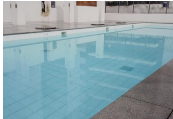
VersiPave®GP enabled level, free draining paving at the swimming pool at the Burswood Casino Apartments in Perth (above).
