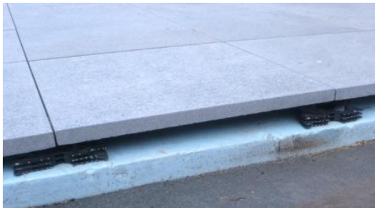
The 1,200m 2 free draining rooftop of Transport House in Sydney (above), with pavers supported on VersiPave®GP positioned on insulation board (below).
